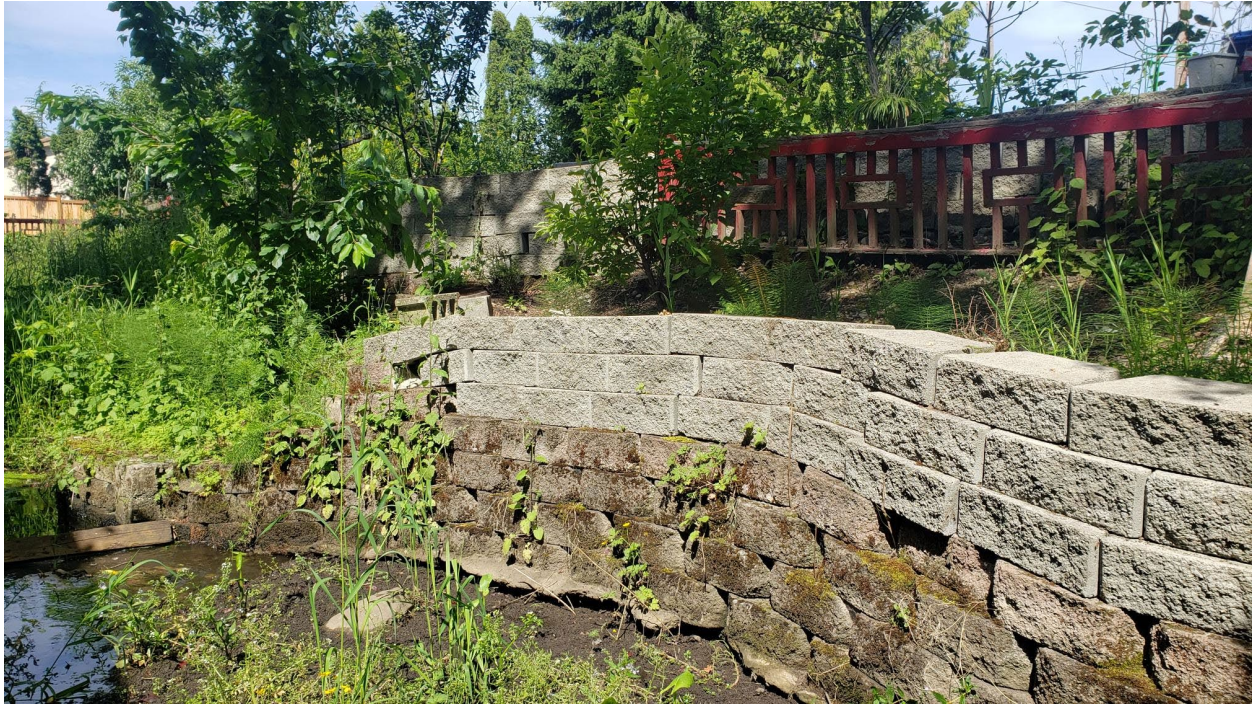
Figure 3. Concrete block wall along stream channel with three new layers and clearly distinguished by discoloration and moss accumulation.
