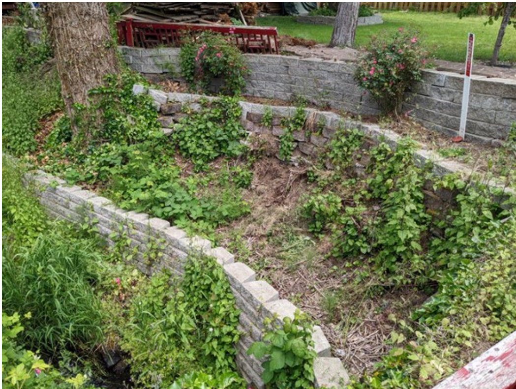
Figure 4. Three levels of concrete block walls including the stream channel, middle level, and upper level. The upper level appears to be of entirely new construction.
